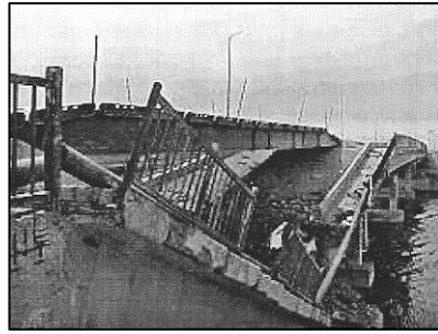
North Ramaylah bridge after
